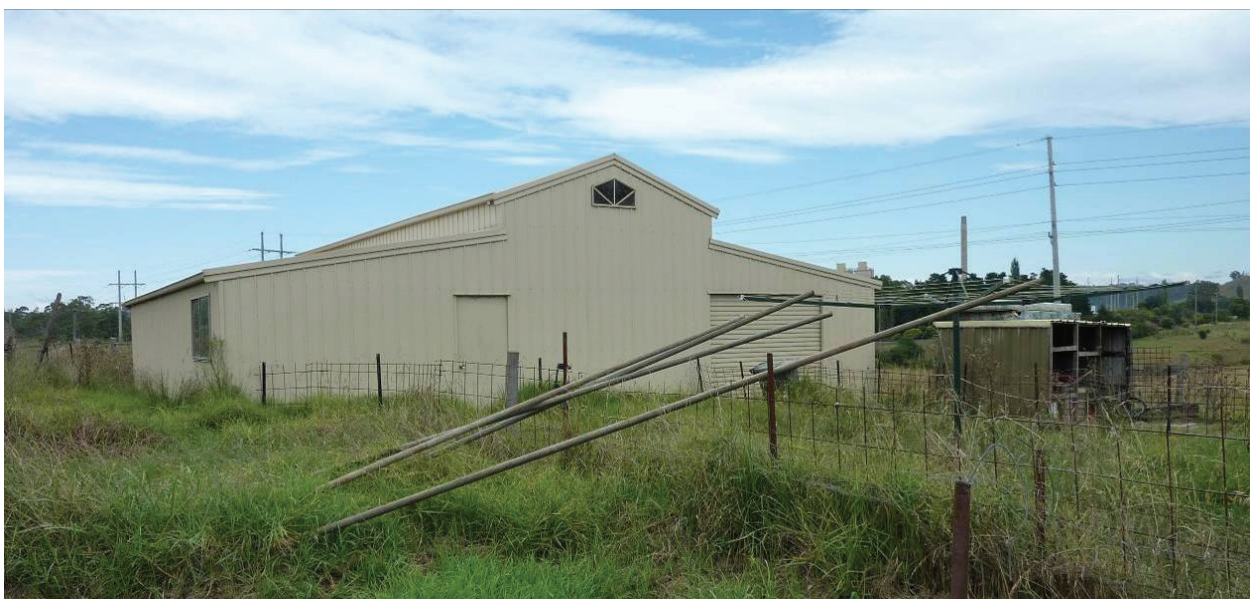
Plate 5.4 Three-Bay Steel Shed at 290 Picton Road
