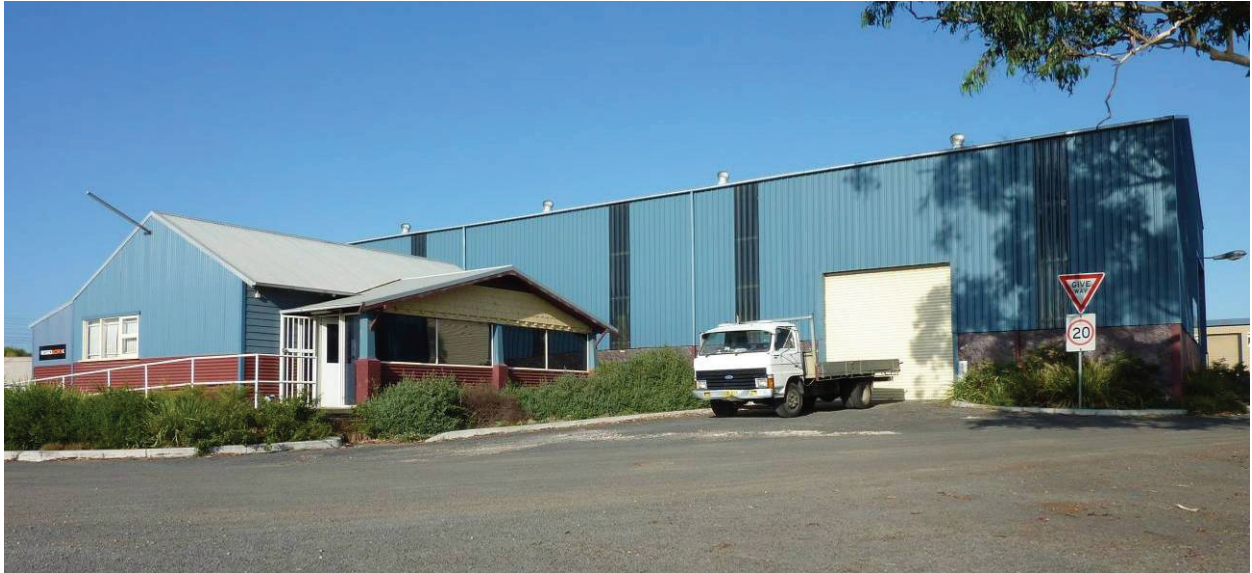
Plate 5.3 Steel Portal Framed Building at 240 Picton Road
