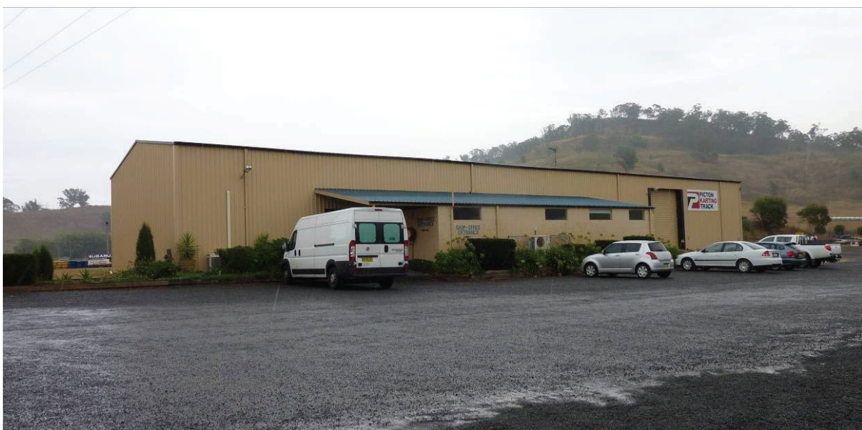
Plate 5.2 Steel Portal Framed Building at the Picton Karting Track
