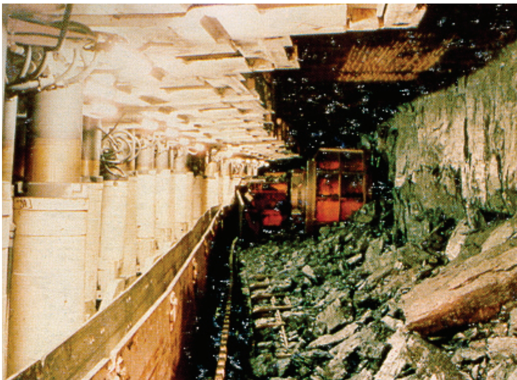
Fig. C.1 Typical Longwall Face Equipment
